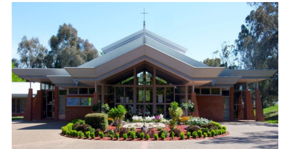
St Michael's Church Tyrrell Cct Kaleen
