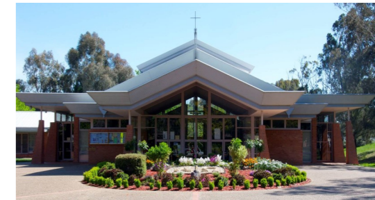
St Michael's Church Tyrrell Cct Kaleen
