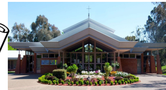
St Michael's Church Tyrrell Cct Kaleen
