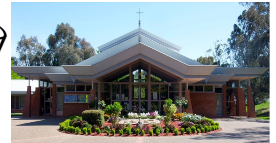
St Michael's Church Tyrrell Cct Kaleen
