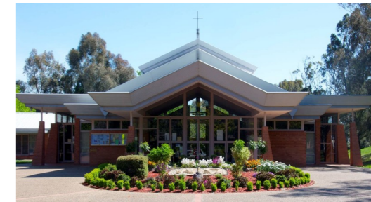
St Michael's Church Tyrrell Cct Kaleen
