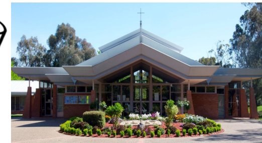
St Michael's Church Tyrrell Cct Kaleen
