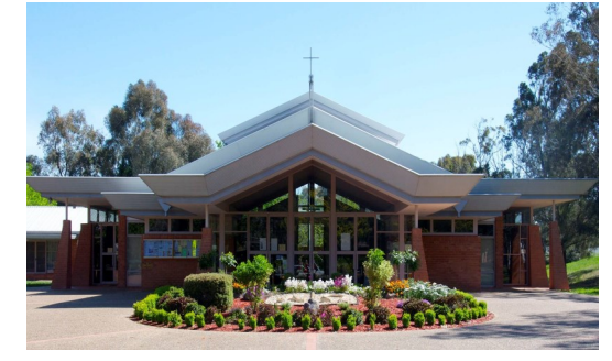
St Michael's Church Tyrrell Cct Kaleen
