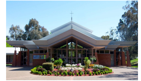
St Michael's Church Tyrrell Cct Kaleen
