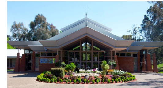
St Michael's Church Tyrrell Cct Kaleen
