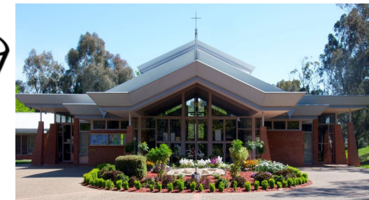
St Michael's Church Tyrrell Cct Kaleen
