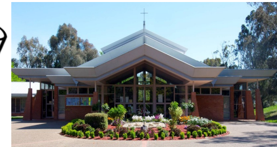
St Michael's Church Tyrrell Cct Kaleen
