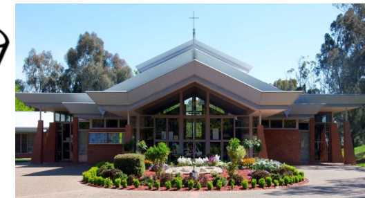
St Michael's Church Tyrrell Cct Kaleen
