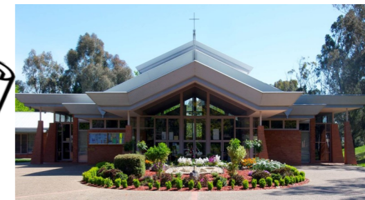
St Michael's Church Tyrrell Cct Kaleen
