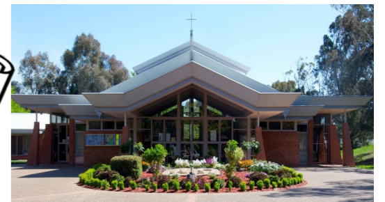
St Michael's Church Tyrrell Cct Kaleen
