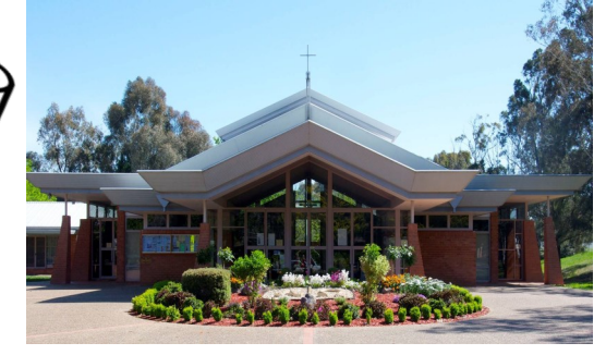
St Michael's Church Tyrrell Cct Kaleen
