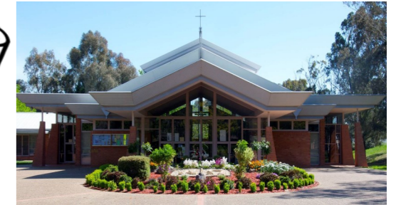
St Michael's Church Tyrrell Cct Kaleen
