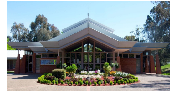
St Michael's Church Tyrrell Cct Kaleen
