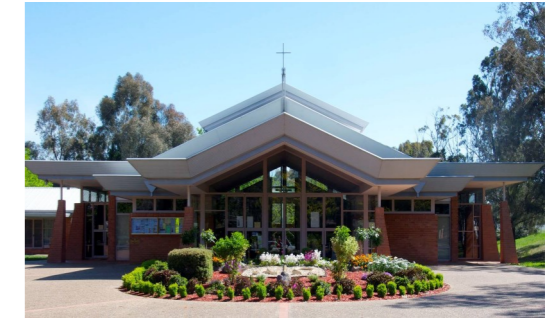
St Michael's Church Tyrrell Cct Kaleen
