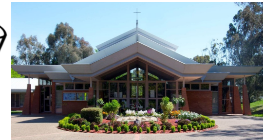
St Michael's Church Tyrrell Cct Kaleen
