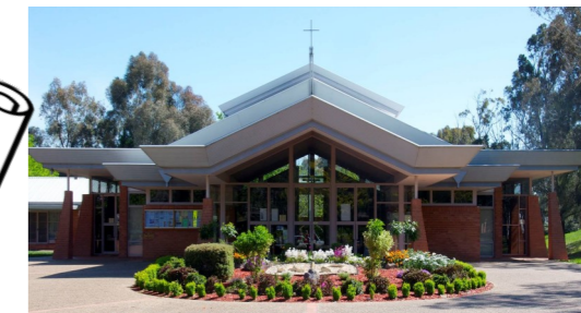
St Michael's Church Tyrrell Cct Kaleen
