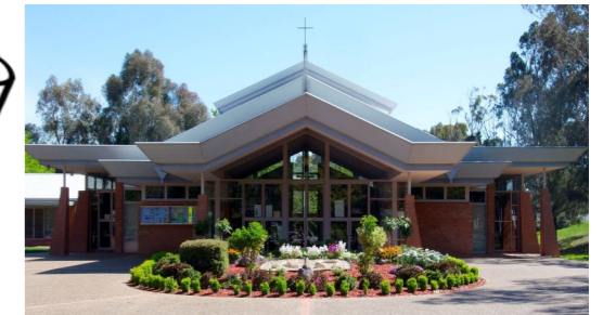
St Michael's Church Tyrrell Cct Kaleen
