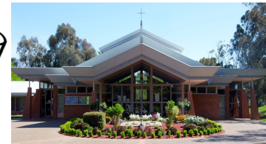
St Michael's Church Tyrrell Cct Kaleen
