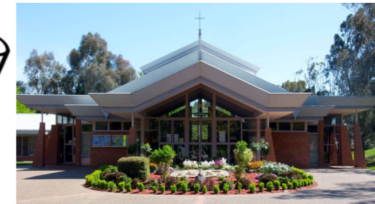
St Michael's Church Tyrrell Cct Kaleen
