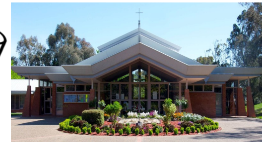
St Michael's Church Tyrrell Cct Kaleen
