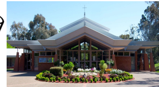
St Michael's Church Tyrrell Cct Kaleen
