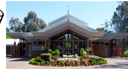
St Michael's Church Tyrrell Cct Kaleen
