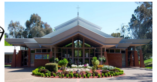
St Michael's Church Tyrrell Cct Kaleen
